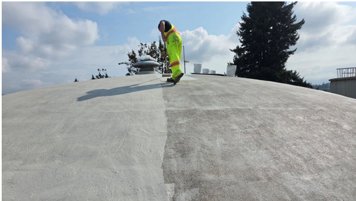
IMAGE | RESERVOIR C EXTERIOR ROOF SEALING.
