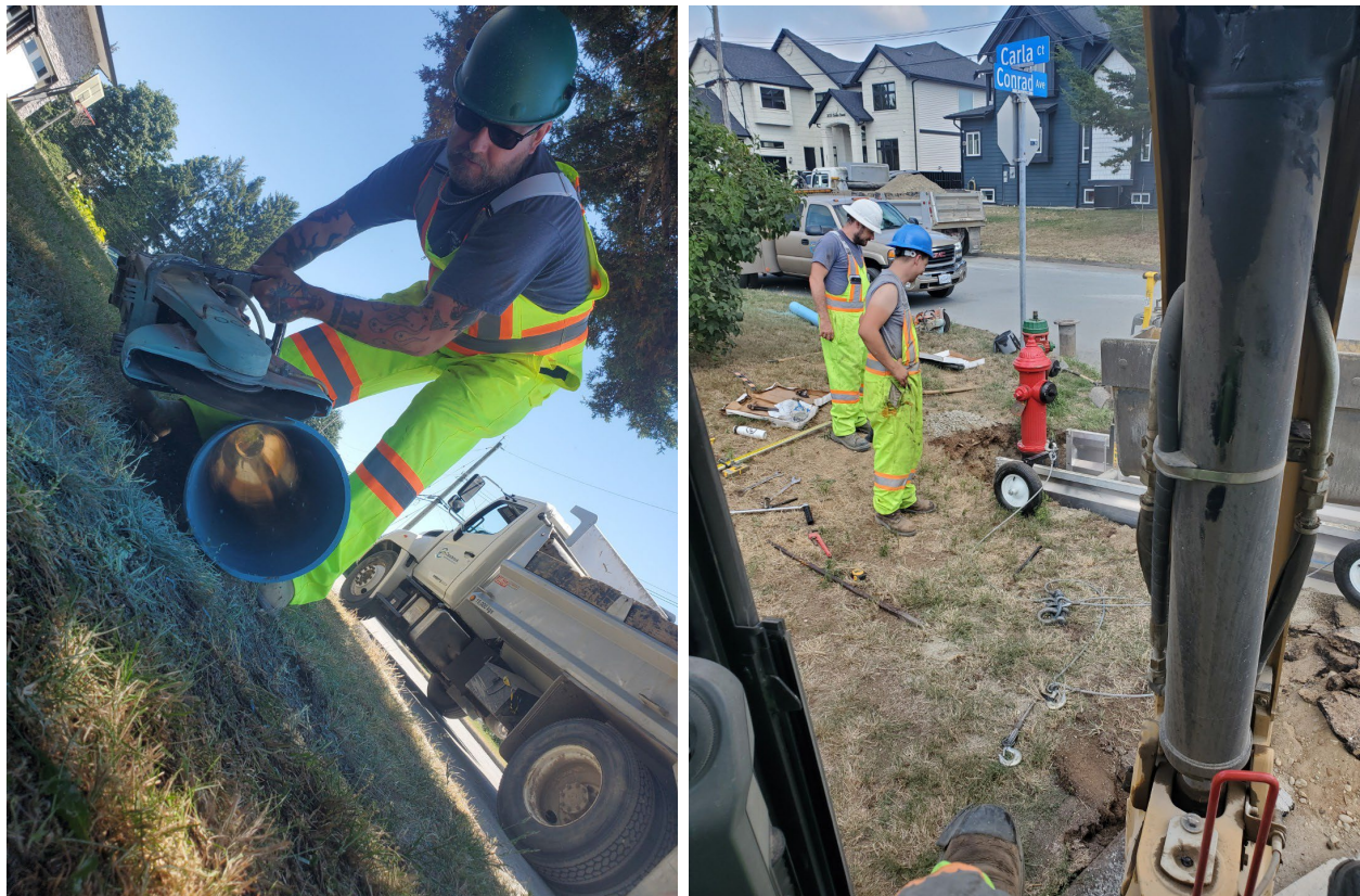
IMAGE | 2024 PIPE REPLACEMENT AND FIRE HYDRANT INSTALLATION ALONG CONRAD AVENUE AND CARLA COURT.
