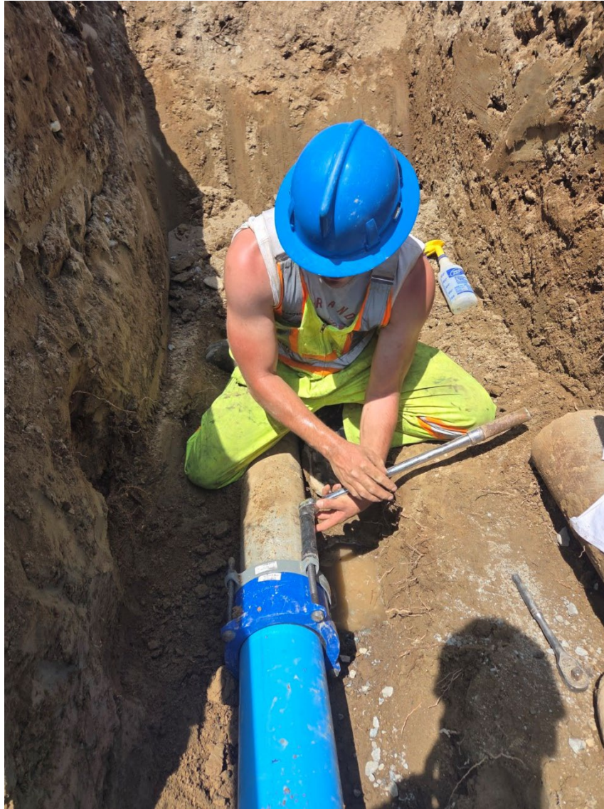
IMAGE | AC CUTOUT FOR SANITARY CROSSING AT 2491 LYNDEN STREET.
