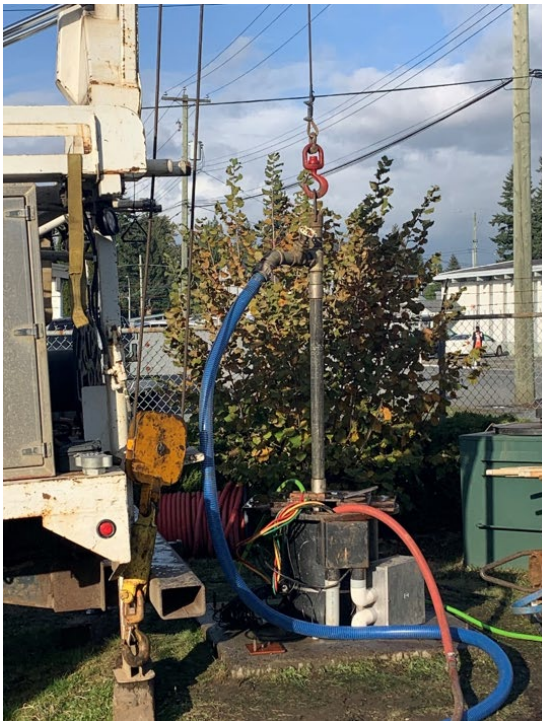
IMAGE | WELL PREVENTATIVE MAINTENANCE FOR RW 2-63/17 IN PROGRESS; FLUSHING IS CARRIED OUT TO REMOVE SEDIMENTS AND DISLODGED AND DISSOLVED INCRUSTATIONS (MOSTLY IRON SCALING) FOLLOWING THE APPLICATION OF ACID DESCALER.
