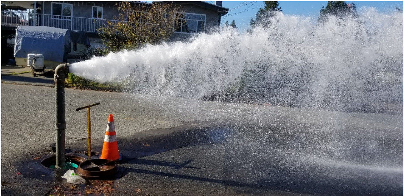
IMAGE | WATER SYSTEM FLUSHING IN PROGRESS.
