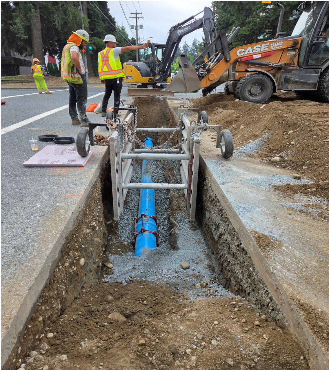
IMAGE | WATER MAIN REPLACEMENT ALONG 2935 CLEARBROOK ROAD - 250-MM BIONAX® PIPE WAS INSTALLED (2025 TENDERED CAPITAL PROJECT).
