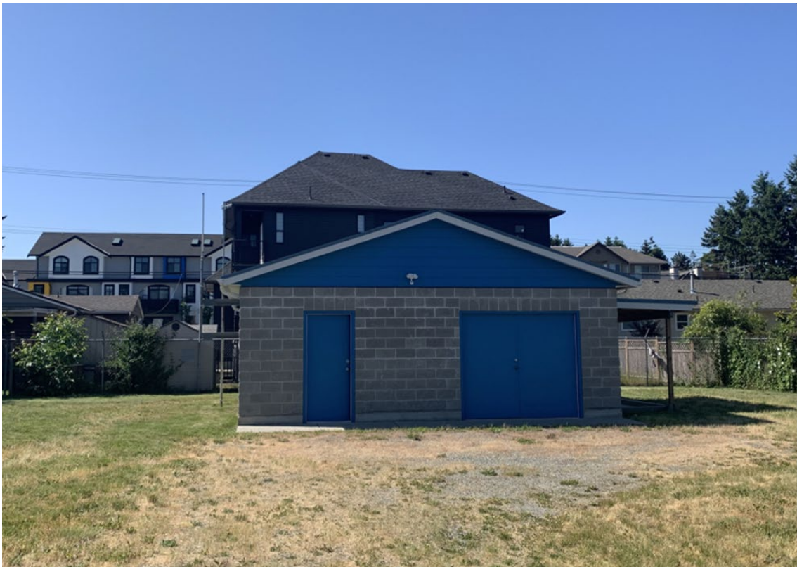
IMAGE | AUTUM WELL FIELD PUMP HOUSE.
