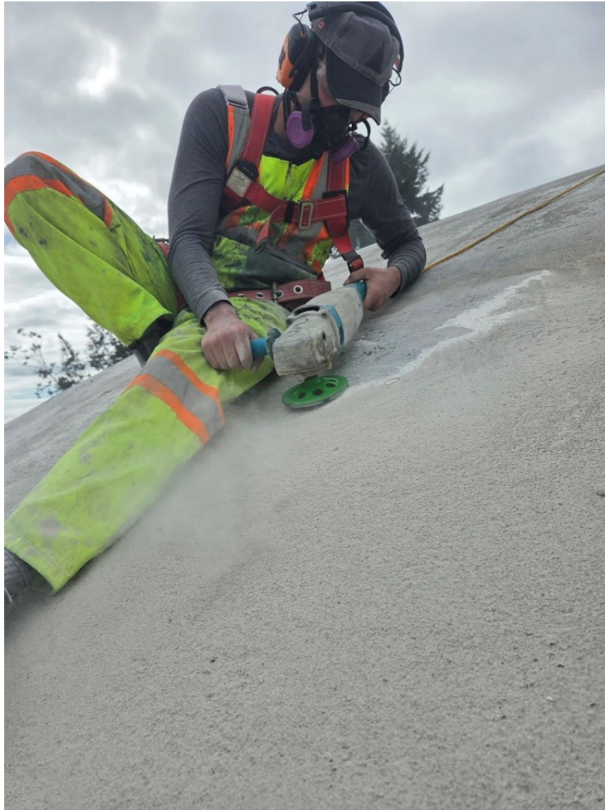
IMAGE | RESERVOIR C EXTERIOR ROOF SEALING – SANDING OF SELECTED SECTIONS OF THE ROOF (WHERE FILL WAS APPLIED) PRIOR TO COMPLETE ROOF SEALING.
